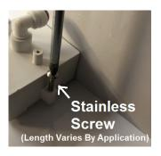
marine-grade sealant is used on the tip of screw. Warning: If your screw is too long it may puncture your hull. Always make sure your screw length is correct.
